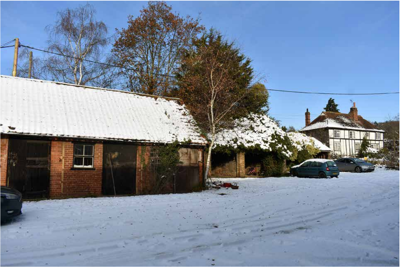
Plate 7: Outbuildings on the north side of the farmyard at Hole Farm, looking north-east
