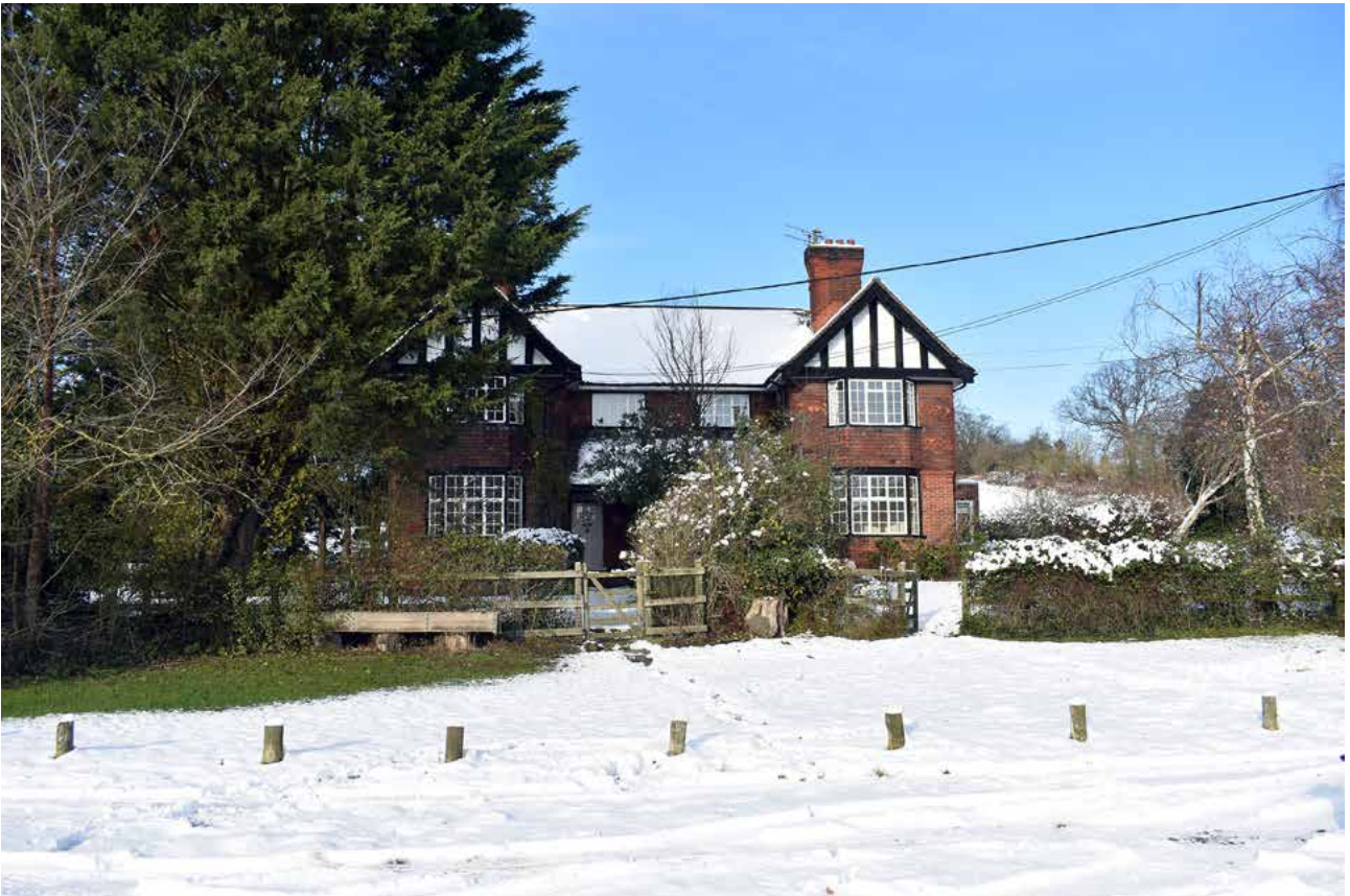
Plate 6: The cottages at Hole Farm, looking north-west
